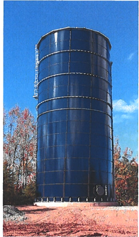
The Pugwash water reservoir is 60' high and has a capacity of one million litres or about three days' supply of water. It can be seen from the road at Port Phillip.
